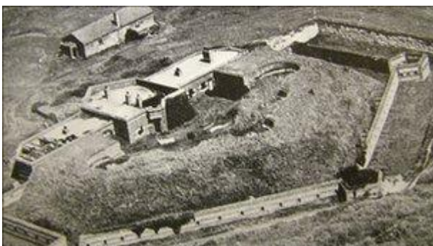
An aerial view of Littlehampton fort, showing the ramparts, Carnot wall and vertical counterscarp.
