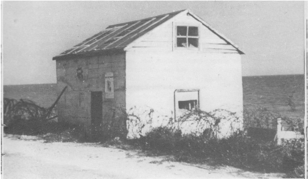
A disguised block-house on the foreshore off Harsfold Road. (Photo: B. P. V. Elsdon).
