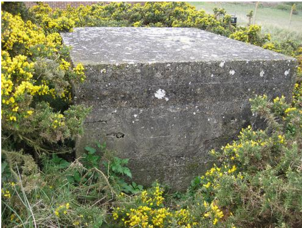
West Beach -small pillbox with corner embrasure, part of a larger bunker.© Michael Fairbrother
