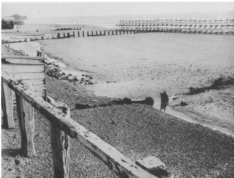
Scaffolding poles on Bognor beach. 7
