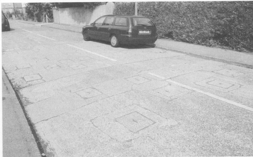
15 Anti-tank hairpin rail sockets in the road surface at the entrance to Townsend Crescent, Littlehampton (TQ 0355 0283)
